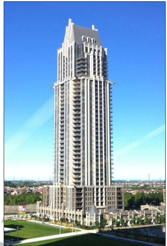
Figure 10: Tall buildings in Downtown Core will be massed in the form of the podium, middle shaft/tower and top.
